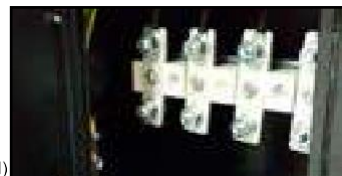
Earth Connection Plug (inner side Control Panel)
